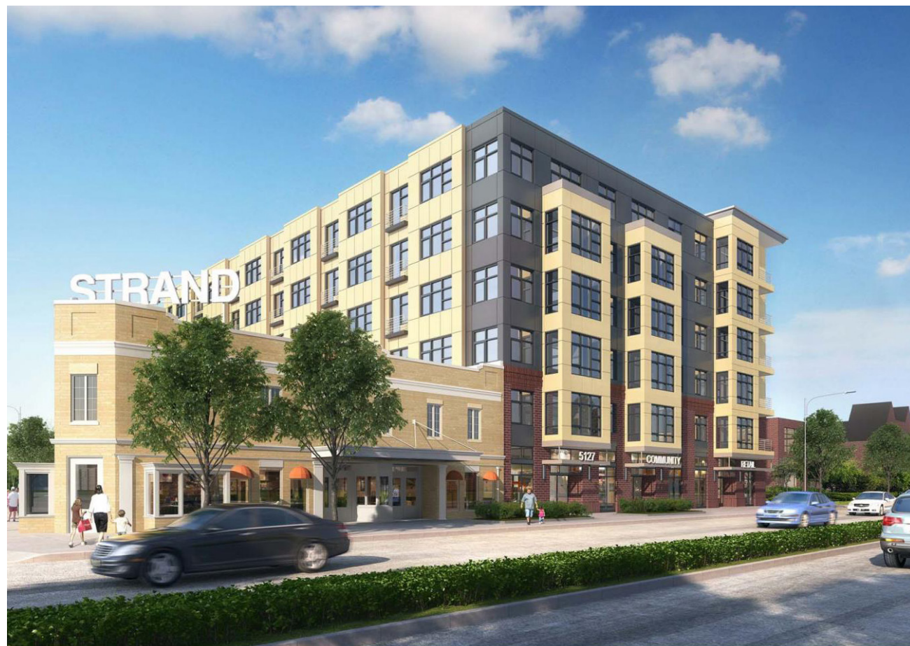
Restored Strand Theater and Strand Residences
